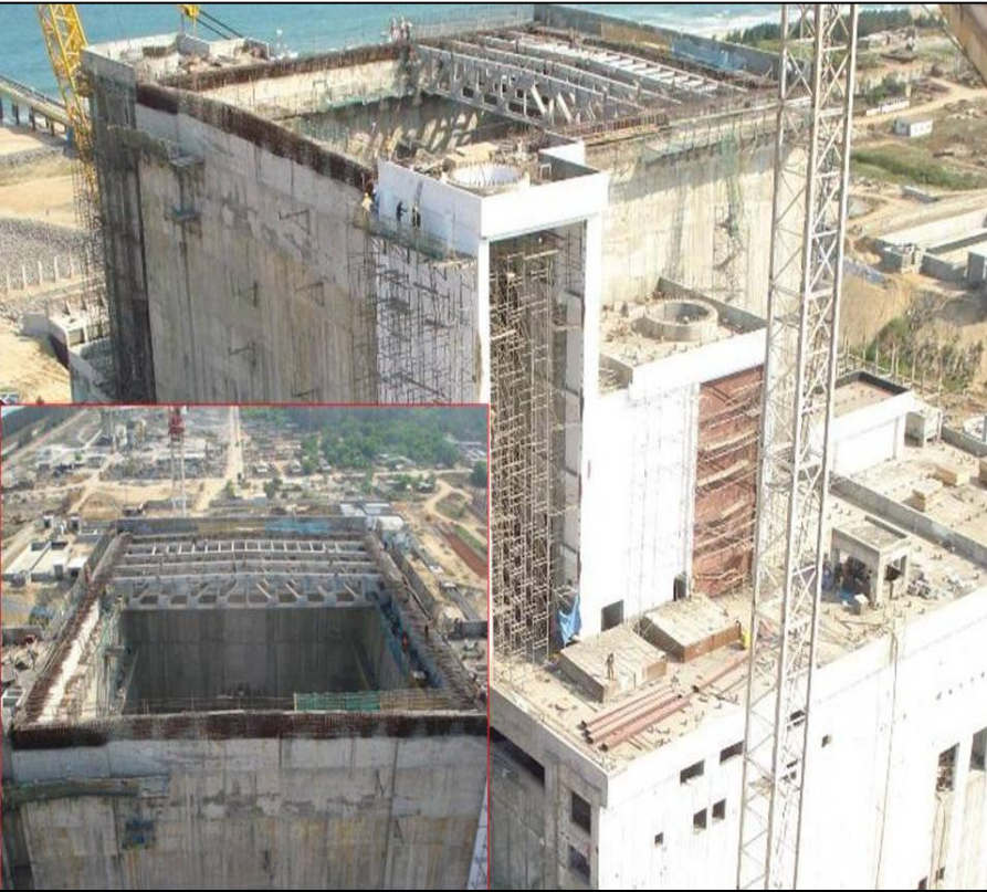
RCB Roof Truss construction
