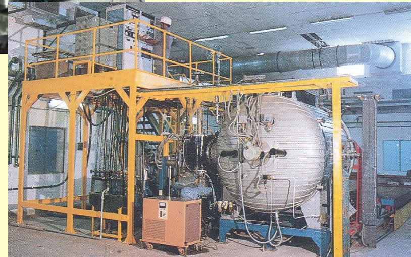
Vacuum Baking Furnace for Graphite coating of PHWR Fuel Tubes
